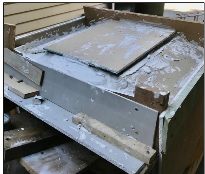
Gib sheet used for strengthening
