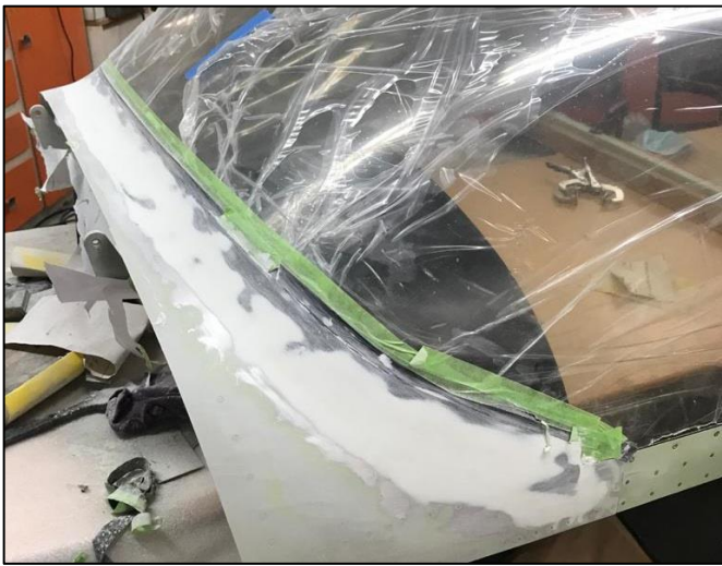
Ready for sanding.
